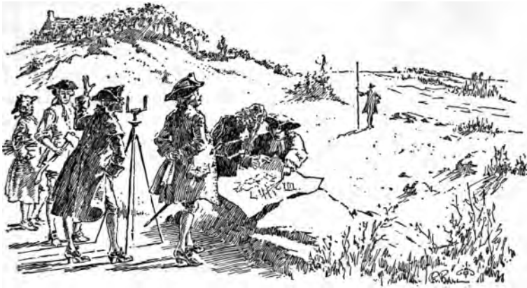
SURVEYORS LAYING OUT BALTIMORE
